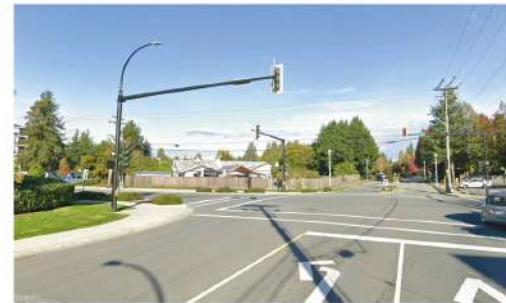
E 208th STREET LOOKING NORTH
