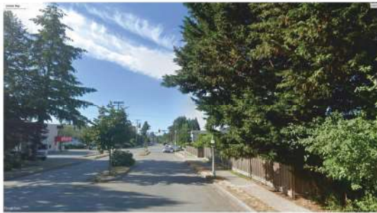
B 208th STREET LOOKING SOUTH
