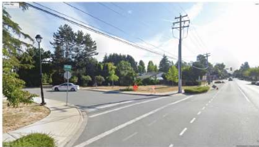
C 56th AVENUE LOOKING EAST
