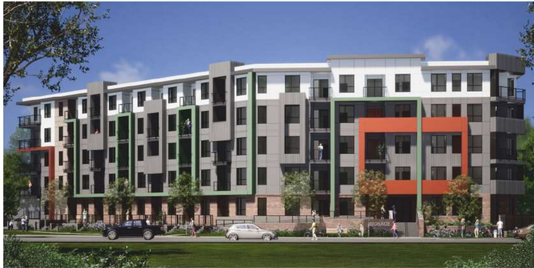
SOUTH/WEST CORNER OF DEVELOPMENT
