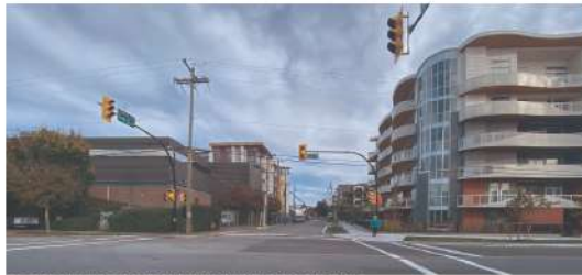
4 - 204 STREET, LEGACY ON PARK AVENUE ON THE RIGHT
