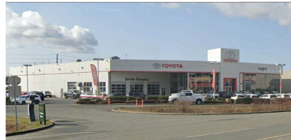
3 - EXISTING VIEW FROM LANGLEY BYPASS
