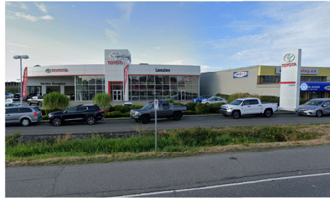
2 - EXISTING VIEW FROM LANGLEY BYPASS
