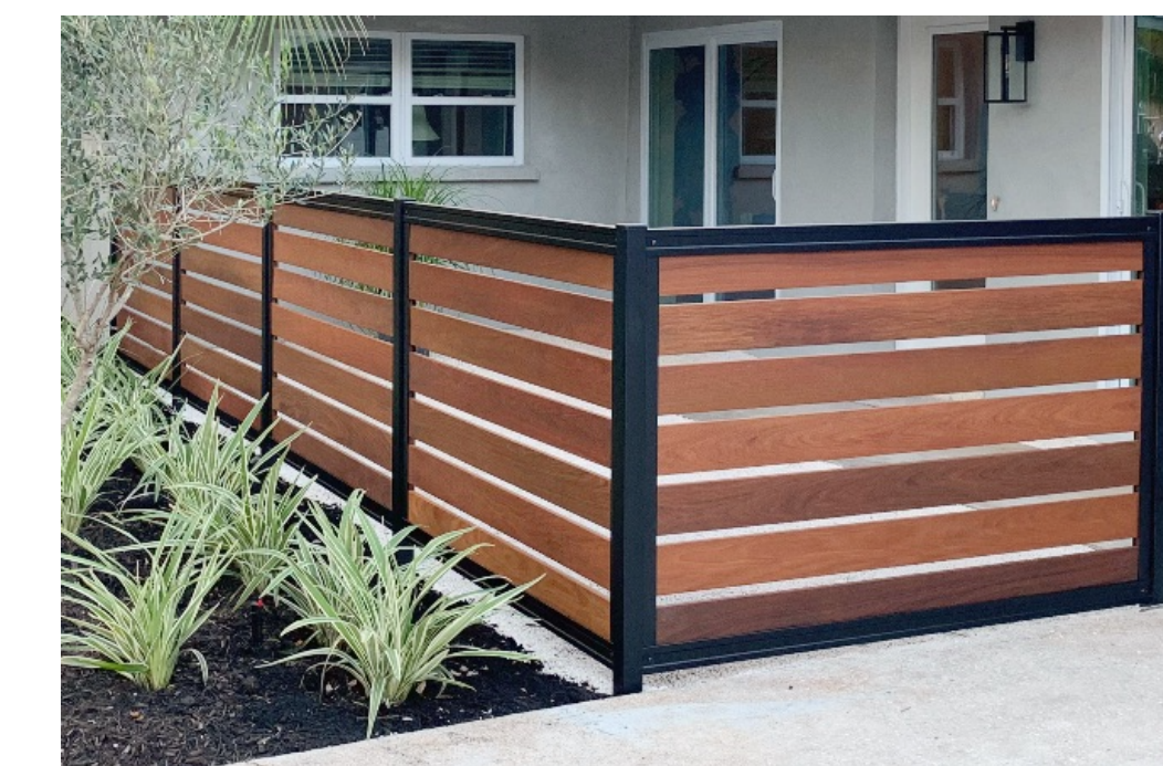
TYPICAL HORIZONTAL SLAT FENCING (COMPOSITE OR ALUMINUM) (NO GAPS IN FENCING FOR ANY ADJACENT PROPERTIES)
