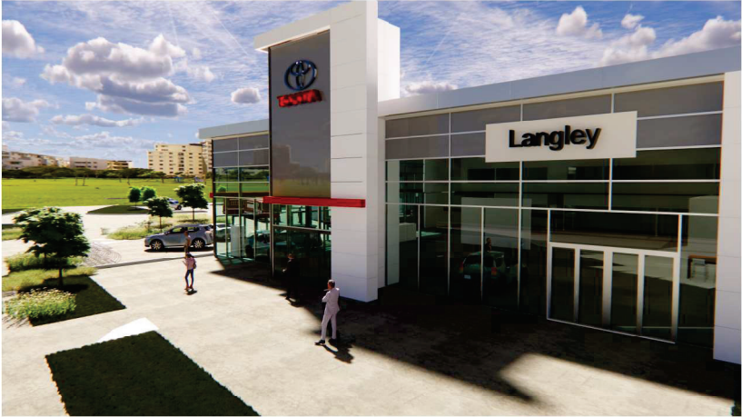
NORTH - WEST VIEW
