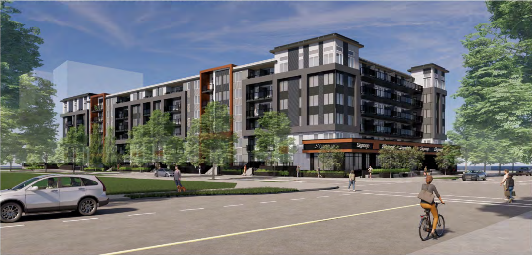
SOUTH/EAST CORNER OF DEVELOPMENT
