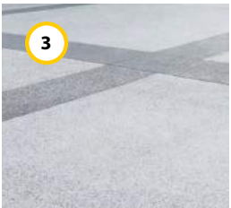
3 Exposed aggregate concrete bands
