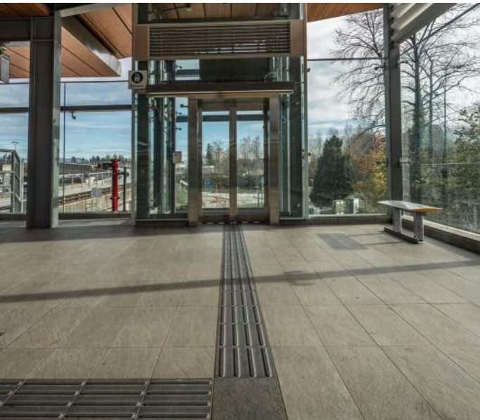
Example of tactile wayfinding tile in contrasting colour, leading to key destination
