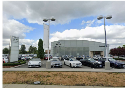
2 - EXISTING INFINITI VIEW FROM COLLECTION DRIVE
