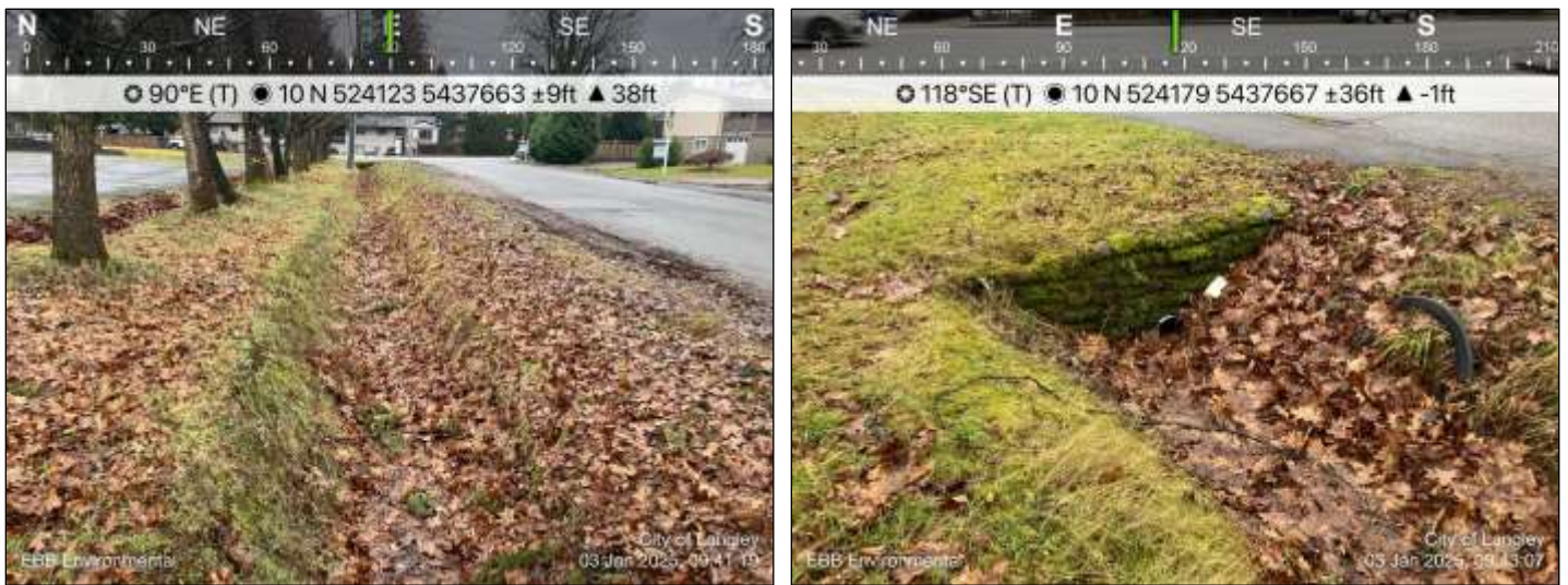
Figure 7. Overview of the aquatic and riparian conditions associated with the watercourse present along the south property boundary (WC-1). Both banks of the watercourse are regularly mowed, and the watercourse was not wetted during the time of the assessment. Narrow culverts (pictured on the right) are present at both the upstream and downstream ends of the section running adjacent to the Project Footprint.
