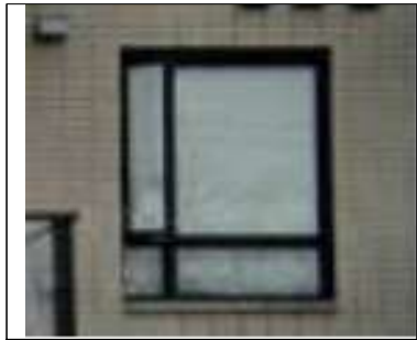
1 - Double Glazed Windows Color to Match: Benjamin Moore Black Ink_2127-20 Glass: Clear
