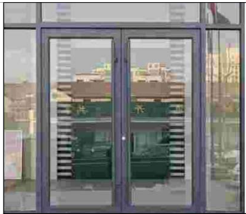
2 - Aluminum Door & Double Glazed Glass Color to Match: Benjamin Moore Black Ink 2127-20 Glass: Clear
